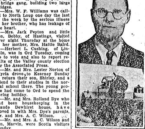
No, this is not a new type cigarette lighter. It's a gasoline engine—only three inches long. The handwork of John Benson, San Francisco machinist, the engine develops about 1-60th of one horsepower, operates normally at 1500 revolutions per minute, weighs two pounds, has 50 working parts and its gasoline tank is filled with an eyedropper.
