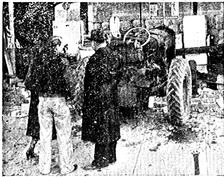
After the city tractor driven by Chief of Police Covert crashed into the plate glass window of the Auble garage Monday morning, doing damage estimated at $400 to $500, this is how the scene looked. In the foreground a Quiz reporter is getting the low-down on the unusual accident from Elwin Auble.—Quiz Photo.
