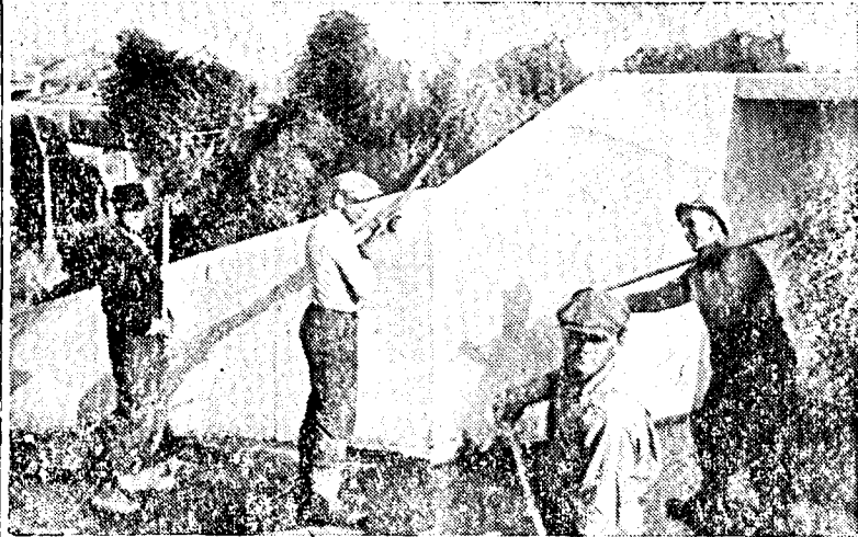
A single day was all the time farmers on the Ord-North Loup canal needed to clean the ditch and get it ready for irrigation, the work being done last Thursday. A group of North Loup business men helped with the work. Russian thistles which blew into the canal during the fall and winter had to be pitched out and burned. Here is seen a group of farmers hard at work near North Loup.—Photo by Birmingham.
