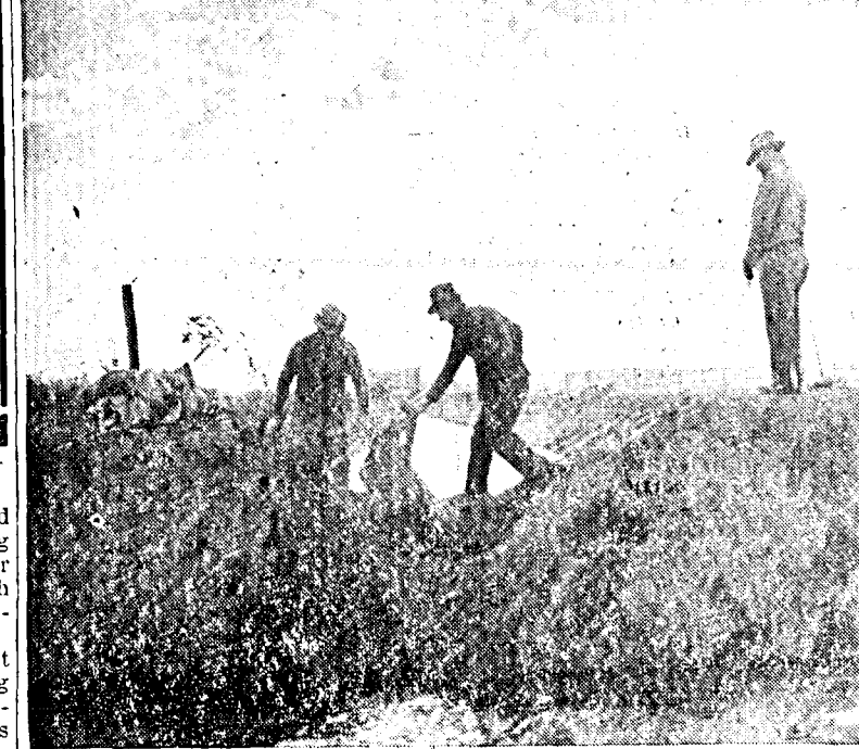
In the upper picture is shown the series of concrete drops constructed at Bassett park as a WPA project with L. Berger as supervisor, this photo being taken Friday afternoon just as water from the Taylor-Ord canal reached the park. A group of city officials and irrigation board employees were on hand to watch the demonstration. But something went wrong a few moments later, as pictured below. An underdrain on No. 11 highway west of the W. H. Barnard home washed out. Here Watermaster Walford and an assistant are shown in an attempt to plug the break with sandbags filled by General Manager Wareham. The attempt was unsuccessful and water had to be shut down above the break. Repairs to the underdrain haven't yet been made so the canal through the park is dry again.
